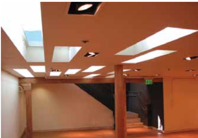
. . . and channeling natural light to open up a previously windowless basement workspace.
